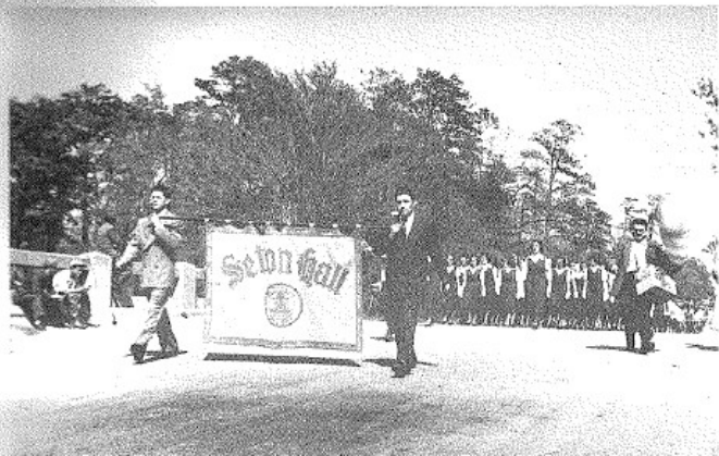
GROUND BREAKING MAY 1949
